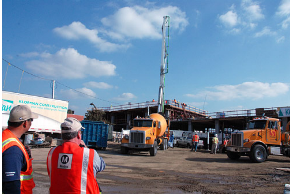
Crew wraps 'last pour' at Metro Atlantic Parking Structure construction site.
